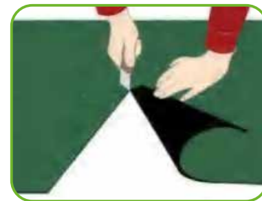
⑦ Cut the artificial grass into the shape desired
