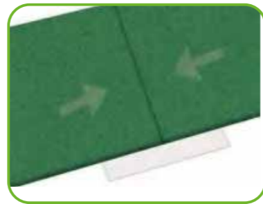
⑥ Press the artificial grass down & fix it
